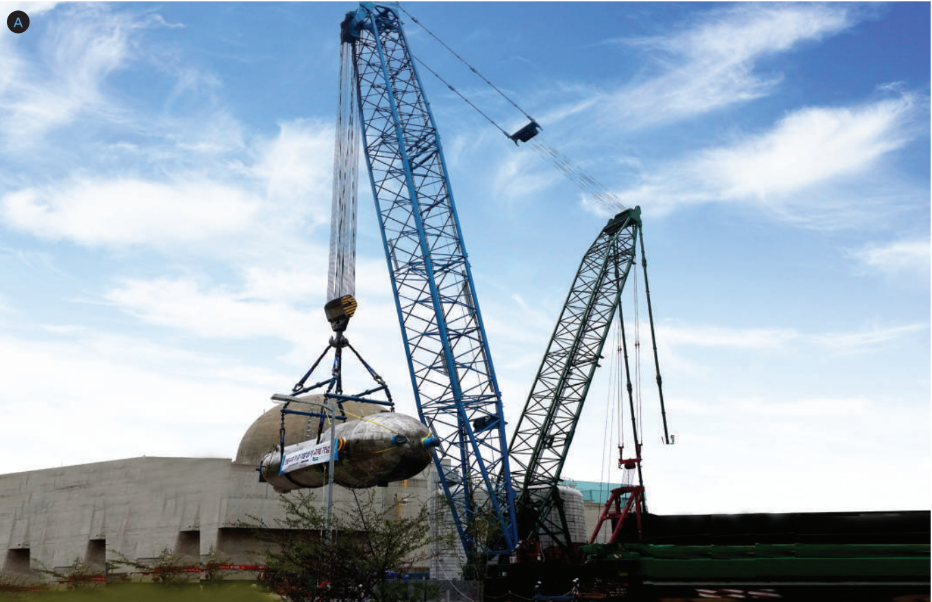
A A | M1200 (1,300T) Installed vapor generator for Ulijn No.4 unit
